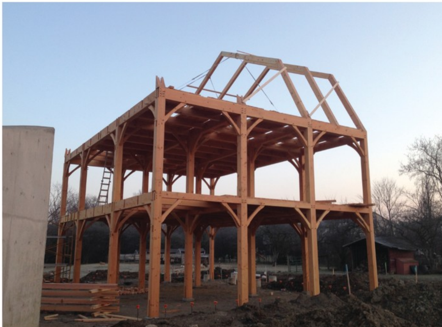
▲ The Real Life Barn presented many design challenges for Timbercraft, including managing increased wind loads, being three stories tall and having a 40-foot clear span gambrel roof system. Photo courtesy of Timbercraft
